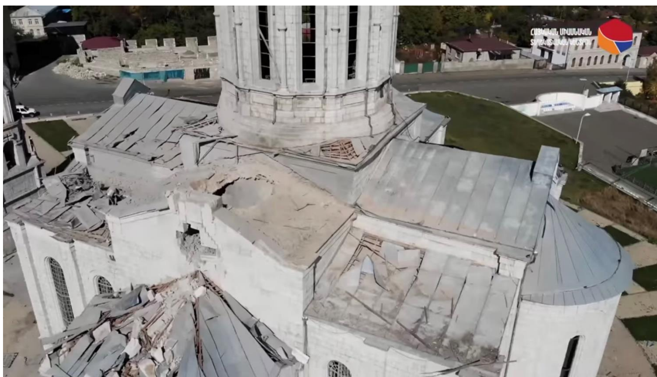
Figure 19: The damaged roof of the St. Holy Savior Ghazanchetsots Cathedral from outside after the second strike
