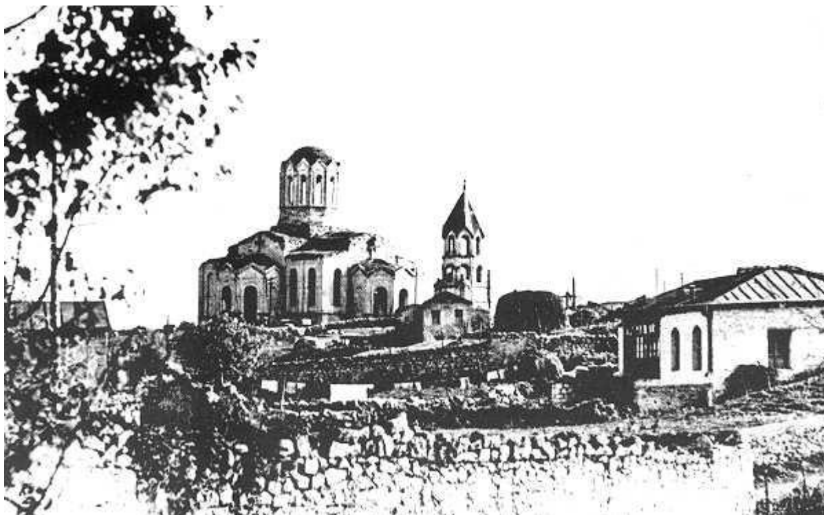
Figures 4 and 5: The damaged dome of the St. Holy Savior Ghazanchetsots Cathedral
