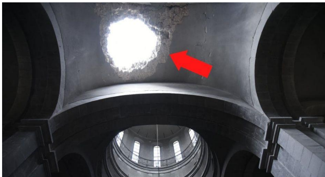
Figure 11: The damaged roof of the St. Holy Savior Ghazanchetsots Cathedral from inside after the first strike
